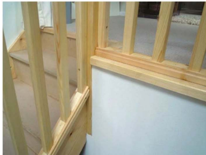
Detail of the stair join to the right
