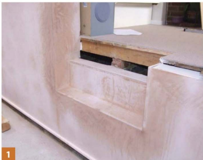
1 Make sure you have created a good 'seating' for the new staircase and measure it up exactly
