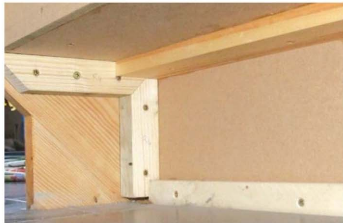
Inner view of the bottom step showing the supports
