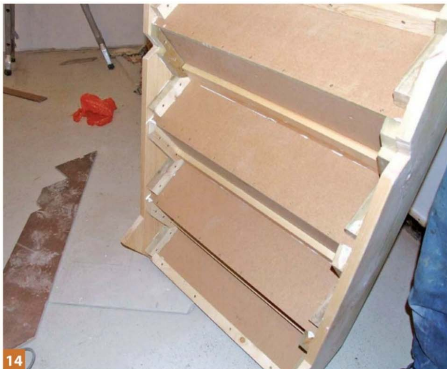
The simple but effective completed construction is visible here
