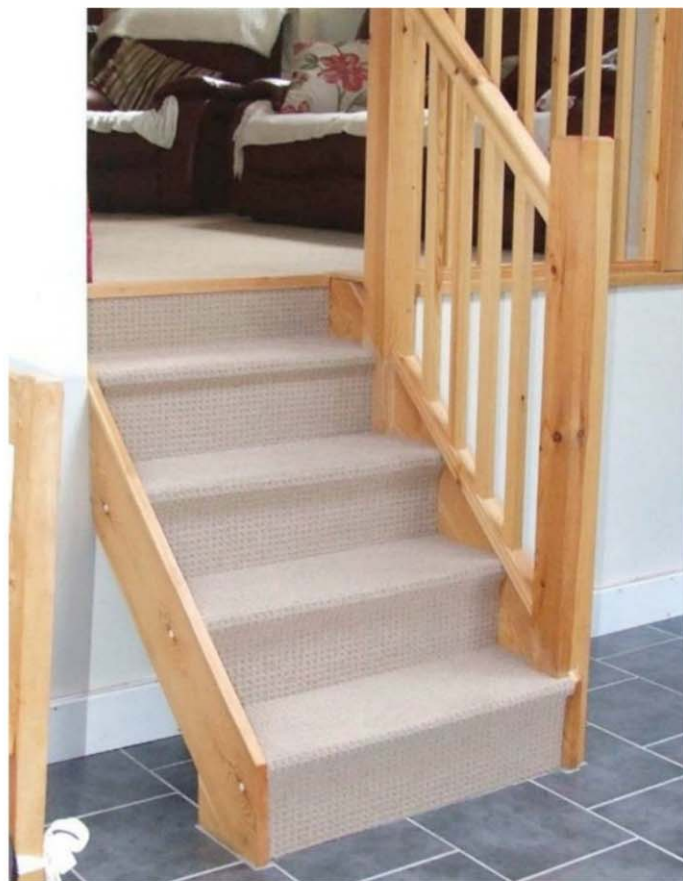
The completed stairs with carpet fitted
