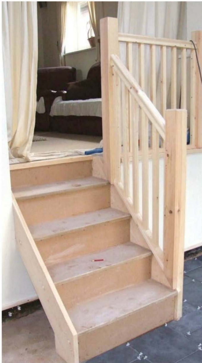
The bottom view of the completed stair assembly
