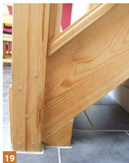
The newel posts are screwed and plugged to the stringer and the plugs trimmed flush
