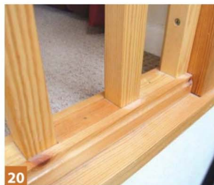
You can make up the balustrade as a separate unit and then carefully fit it between the newels
