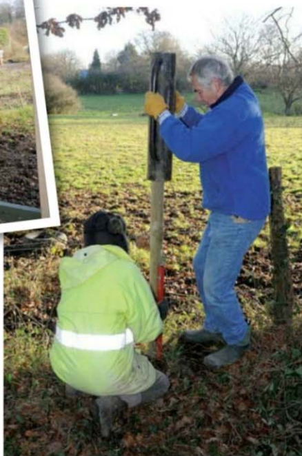
Jim drives a post into the ground with a few mighty whacks from a post driver
