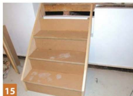
Check for fit and adjust if necessary. Use long screws and plugs to fix it into the surrounding masonry
