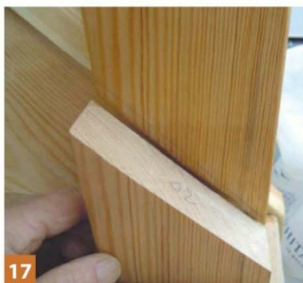
Where the newel post is cut over the stringer refit the waste piece to strengthen the joint
