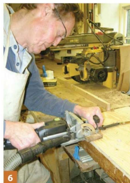
6 Cutting Domino slots in the panel frame
