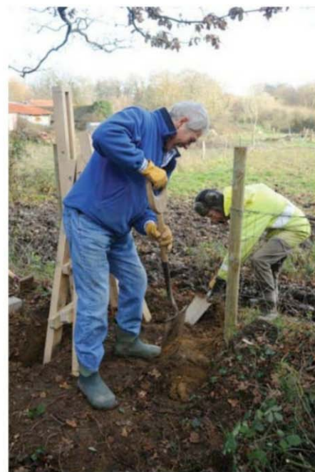
Jim and Giles dig the holes for the stile which will be anchored with angle irons
