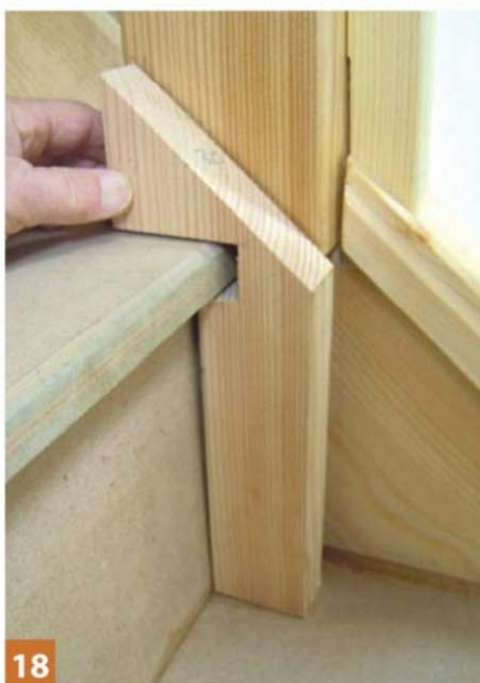
In this case the top post has its waste piece cut to fit around the tread nosing
