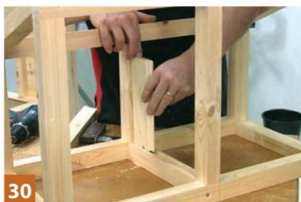
30 You could also use ply for the divider
