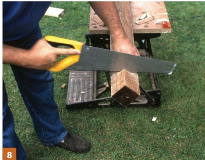
Cutting out the front corner of the post to take the trellis
