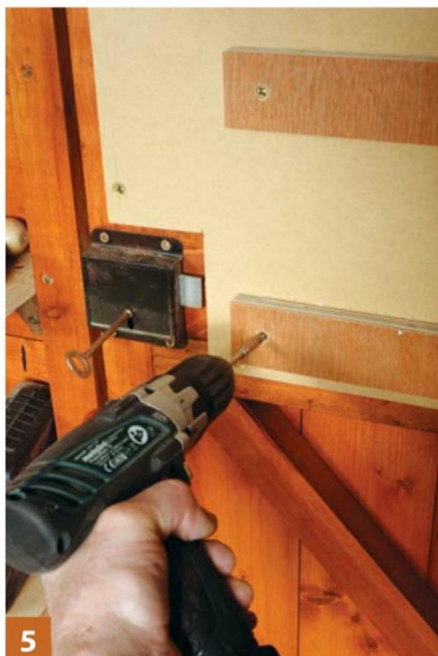
5 I screwed four strips of 15mm ply to the board about 125mm apart
