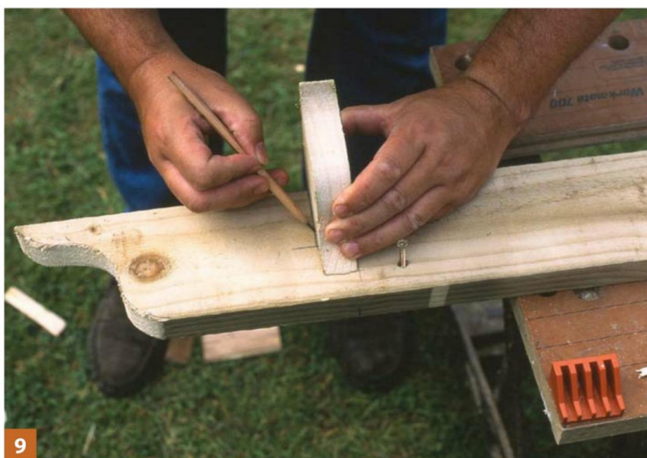
Marking the front beam for cutting out
