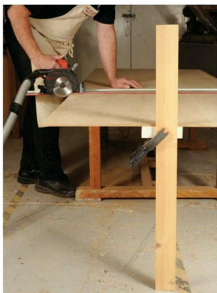
The support leg falls away when the cut is finished
