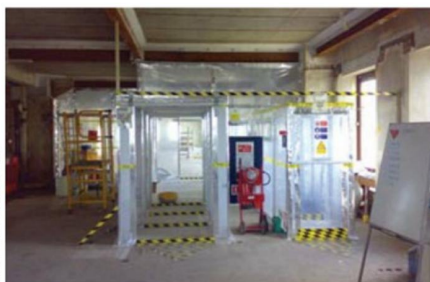
This is a typical asbestos enclosure constructed by Trinitas Contracts in the UK for the removal of asbestos sprayed coating from beams
