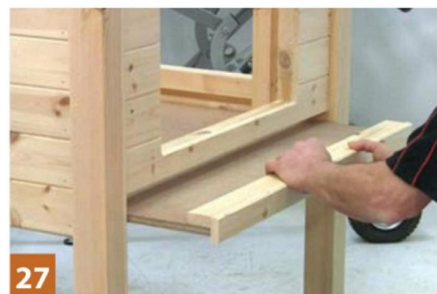
27 Screw a strip of 25 x 50mm onto the top of the base board
