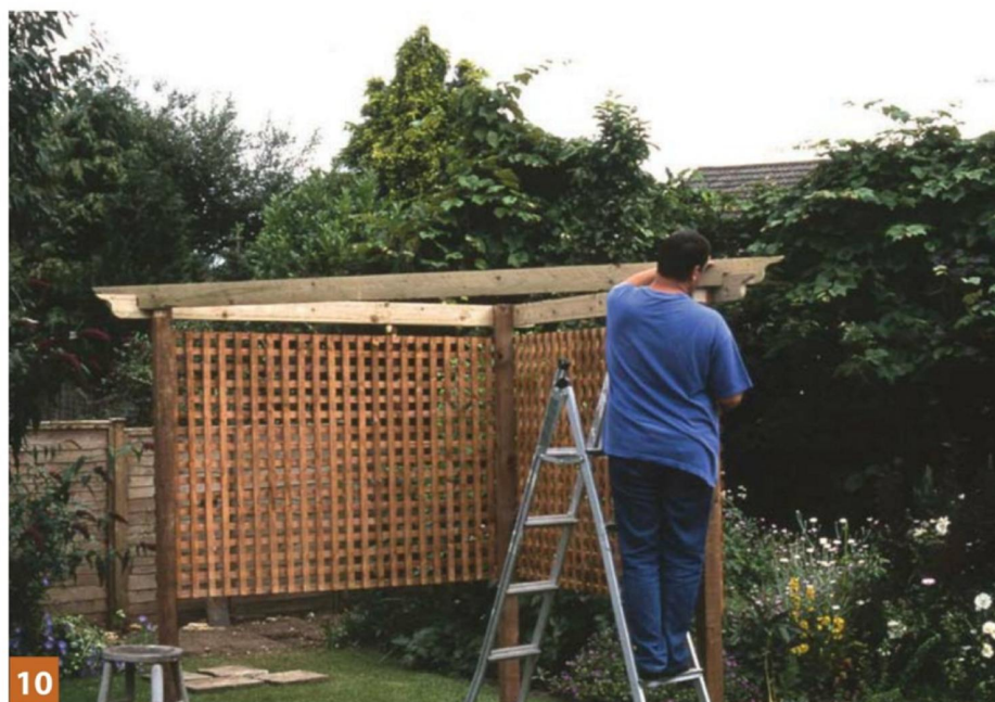
Fixing the front beam in place
