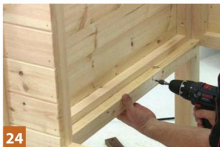
24 Fit the two runners for the base which slides in from the rear
