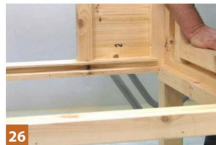
26 Screw the locating strip across the front of the coop
