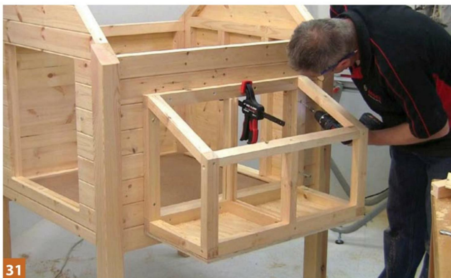
31 Using some Quickgrip clamps, screw the nestbox frame in place
