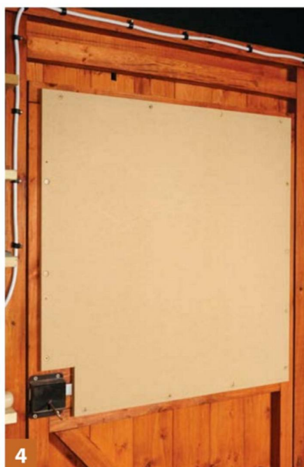
4 I cut some waste pieces of foil wrapped polyurethane foam board to fit behind, before screwing it in place
