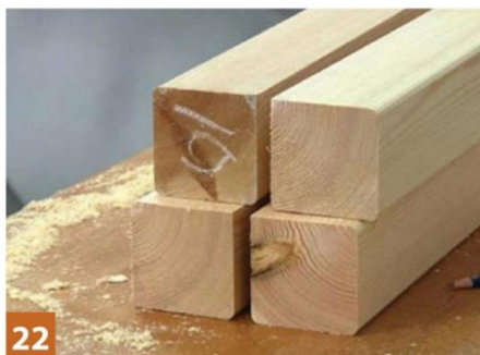
22 Rout a radius on the three exposed corners of the uprights
