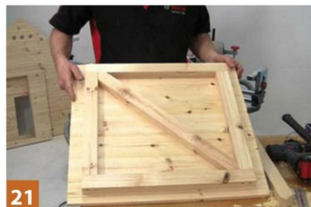
21 The back opening door is another framework clad in tongue & groove
