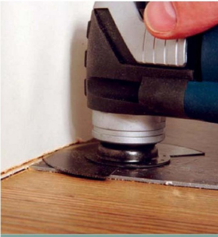
Flush cutting is a piece of cake for the multi-tool
