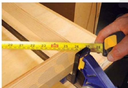
Measure diagonals to check for square
