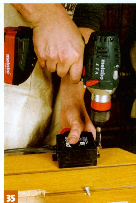
An NVR switch is essential and can be screwed to the underside of the table
