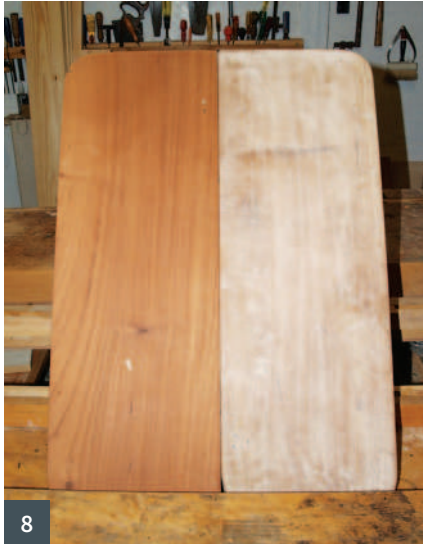
7 The Festool sander did an excellent job of removing the previous sander marks 8 Two flaps side by side. The one on the right is as it arrived; the one on the left is off the Festool 9 Picking the paint out of the rim mouldings. Note the clamp marks from Victorian needlework accessories 10 The three leaves before any colouring 11 Applying grain filler to a leaf 12 The filled leaf left to dry
