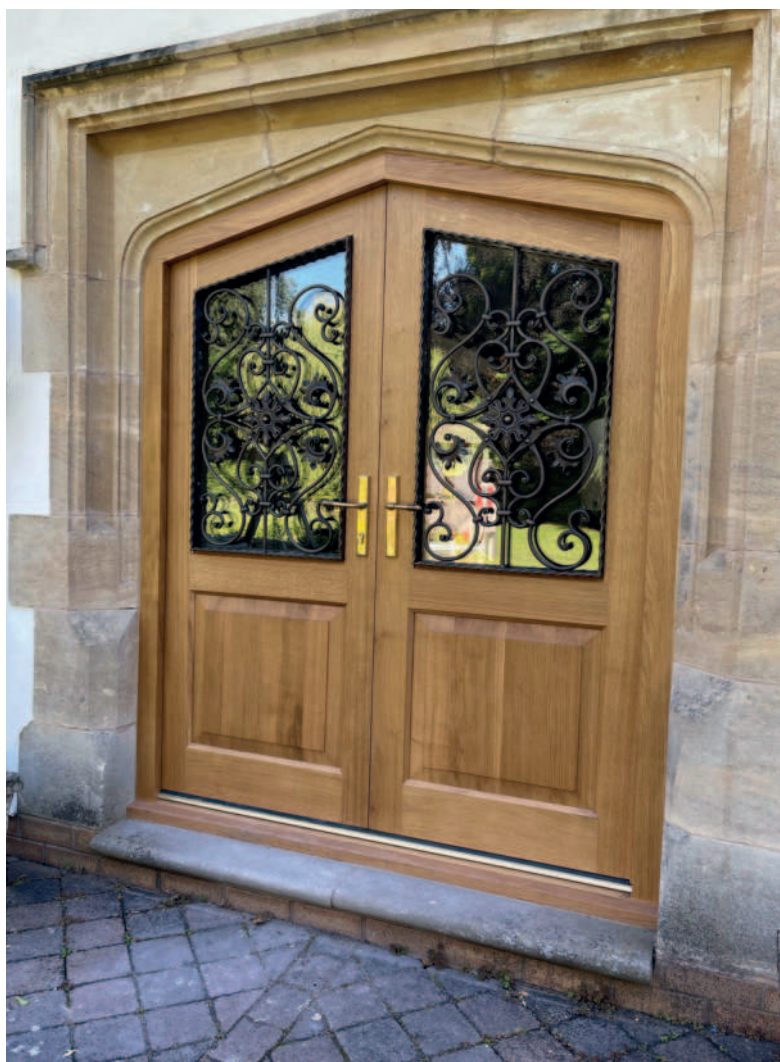
Gothic arched oak double door entrance with bespoke steelwork
