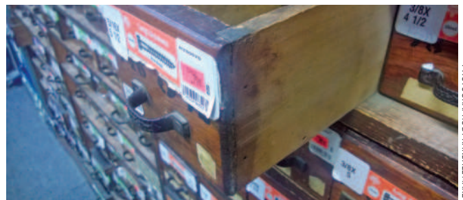
This antique hardware cabinet features drawers made with rebated fronts assembled using nails
