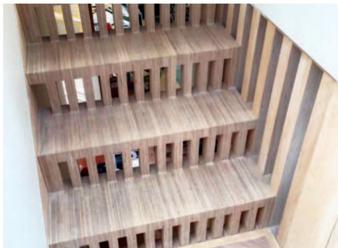
Made for a private home in Wimbledon, this innovative staircase used CNC-cut birch plywood pieces bolted together to form a strong aesthetic statement
