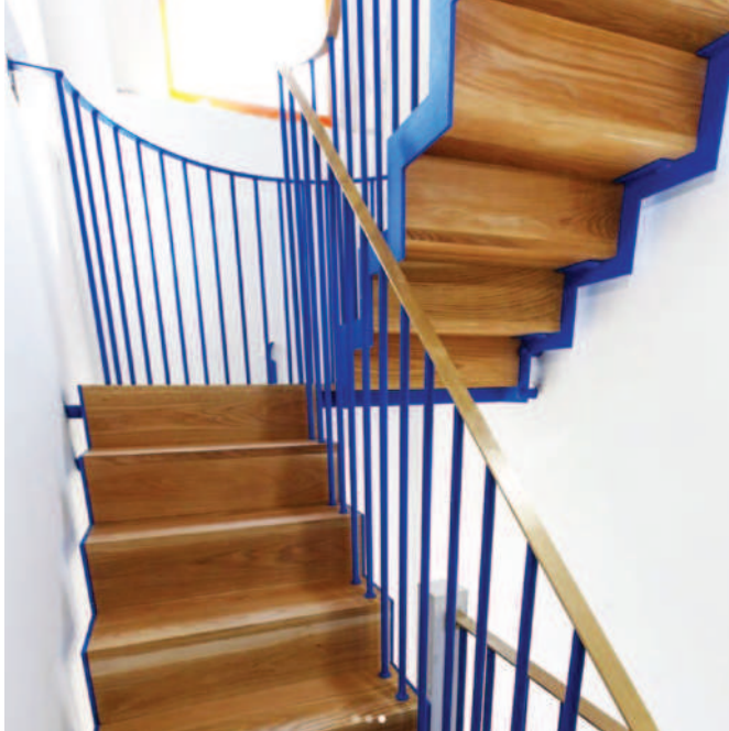
The Blue Stair features a delicate steel framework set off from the out of square walls of this renovated house supports solid oak treads and a brass handrail
