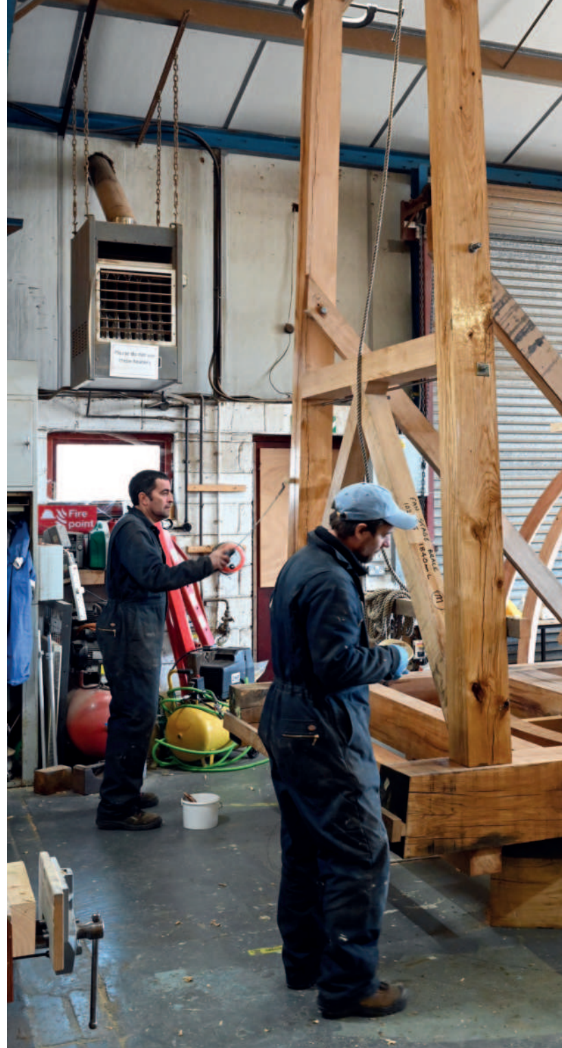
IBTC's commercial team working on the new fantail frame
