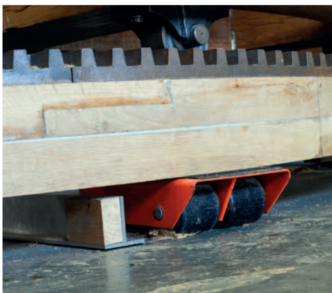
The new curb and bearings for Swaffham Prior
