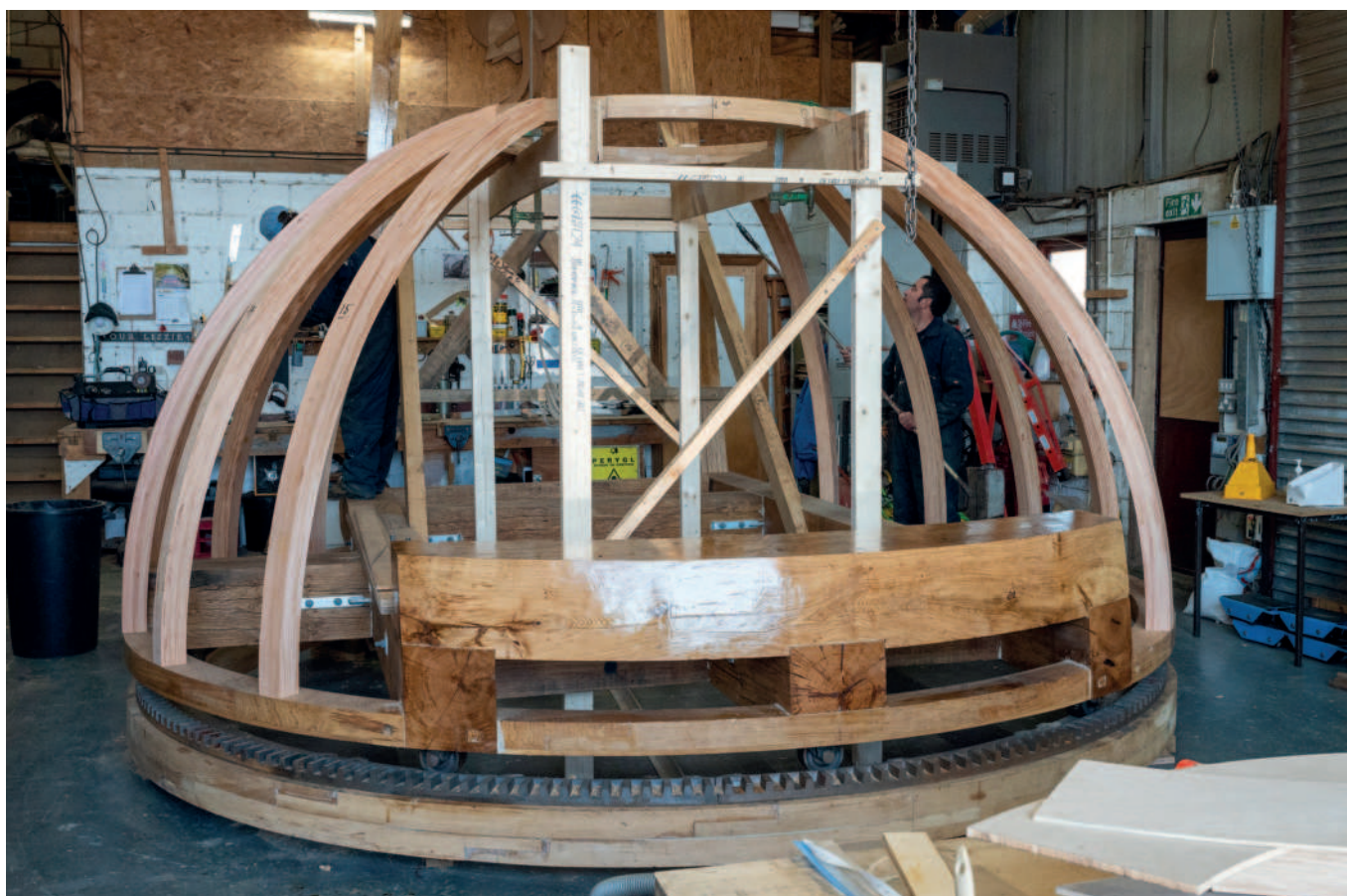
ABOVE: The new cap for Swaffham Prior, with the beam that will support the windshaft OPPOSITE: Swaffham Prior's sister mill at Wicken, showing the Cambridgeshire-style cap
