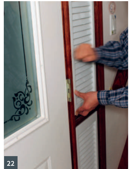
MILLING THE JOINTS: 17 Joining the rails and stiles with a butt joint MAKING THE SLATS: 18 The slats were cut to size 19 Rounding the edges of the slats 20 The edges of the shutter frames can also be rounded ASSEMBLY AND FINISHING: 21 Dry-fitting the slats in the frames 22 Hanging the shutters in place
