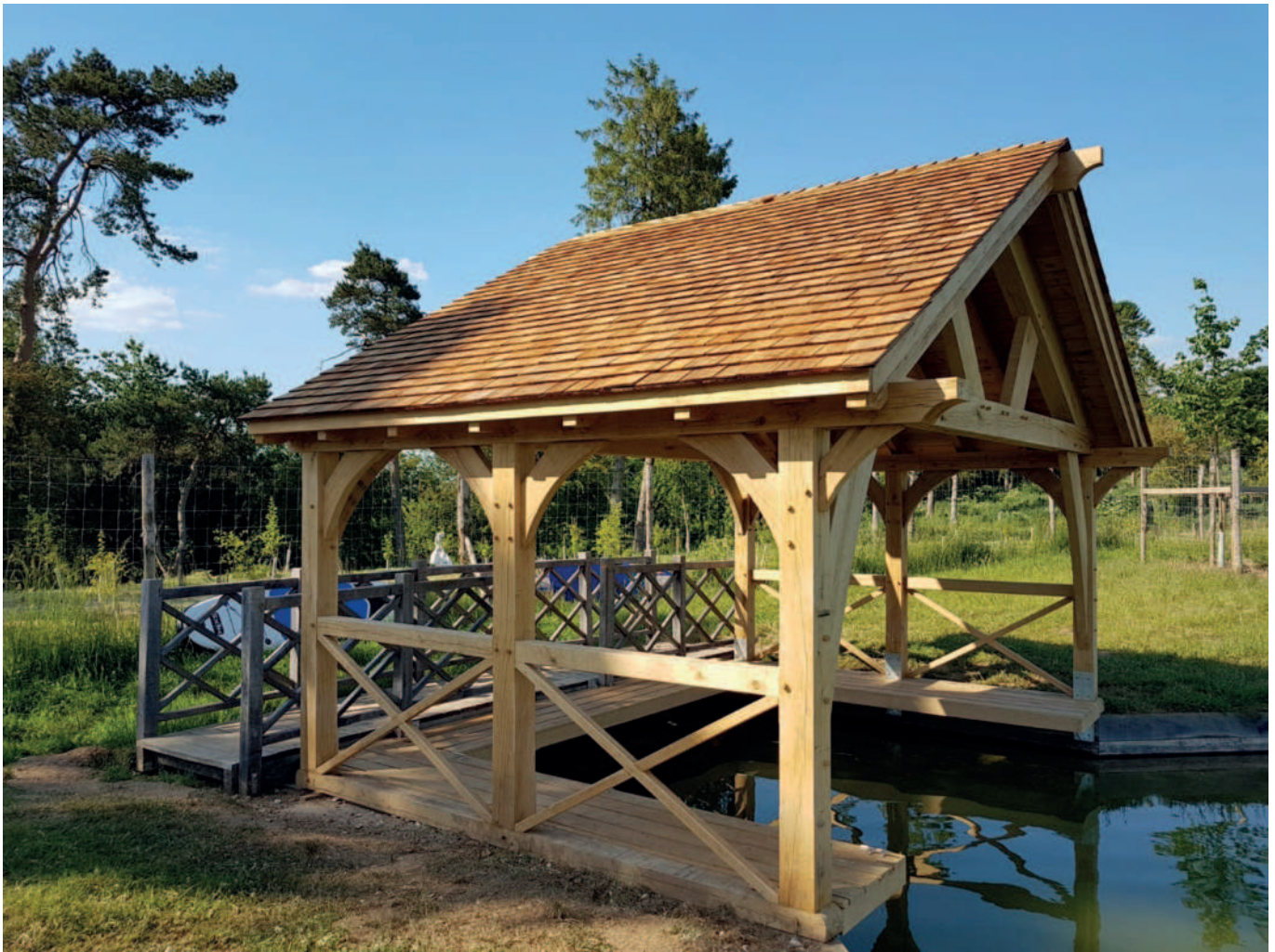
Oak-framed open-sided boathouse with a cedar shingled roof and space in the rafters to store kayaks and canoes
