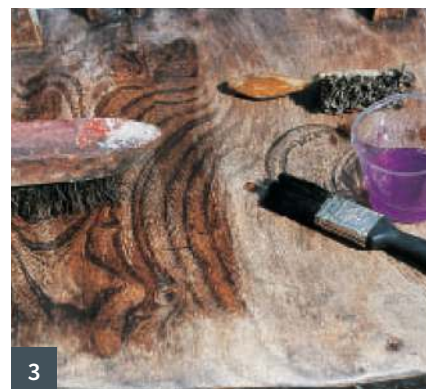
1 Applying a thin coating of stripper 2 Slowly scraping off the old finish 3 Stripping ingrained finish with a wire brush
