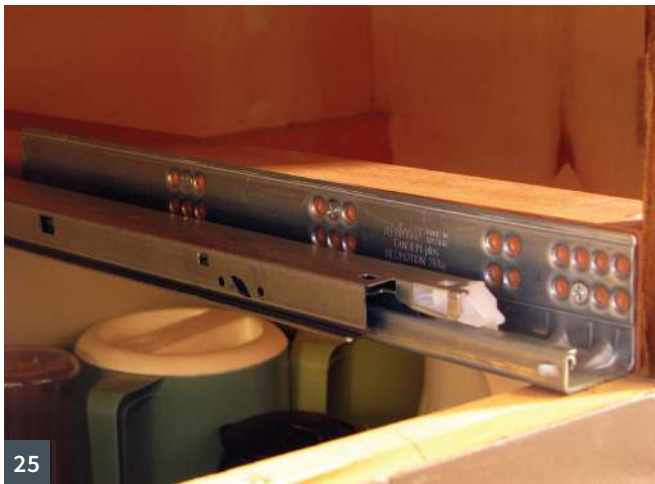
22 A routed slot cut into the top face of the drawer bottoms accommodates the Blumotion slide hardware 23 Testing the fit of the hardware 24 Pulls installed in the six drawer fronts 25 Drawer runner installed inside a drawer pocket 26 Completed drawers run like a dream
