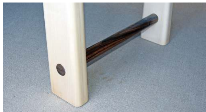
The wedged round tenon detail
