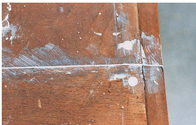
The countersunk screw holes and gap between two of the wood pieces are filled with car body filler
