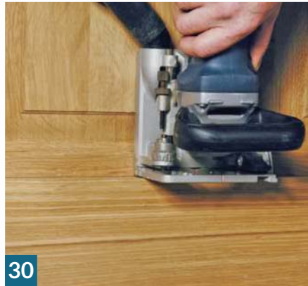
Slotting the top of the skirting board ready to accept a moulding
