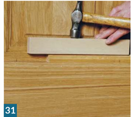
A piece of oak quadrant with biscuit slots is tapped into place using biscuits and glue
