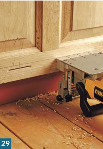
Slotting an oak wall panel to accept matching skirting boards
