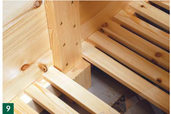
Support for central floor beam, which can be an offcut
