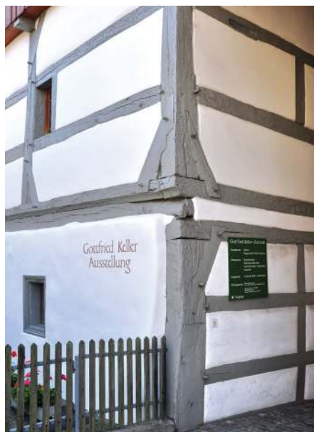
The Glattfelden Bell House, Glattfelden, Switzerland
