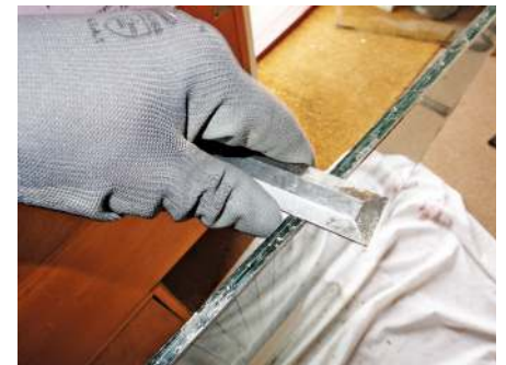
The side of the chisel being used to scrape the edge of a wired glass pane. Note the protective glove
