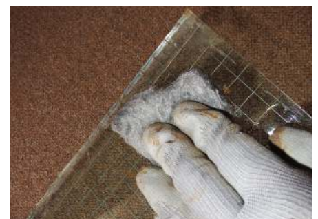
And finally, '0000' wire wool rubbed on the glass to thoroughly remove all traces, including finger grease marks
