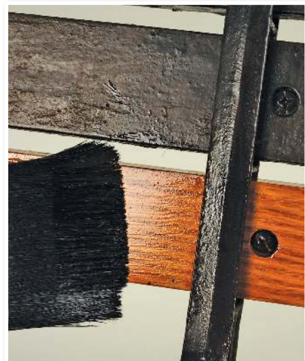
Finally apply a suitable exterior finish such as Sadolin. For teak use teak oil
