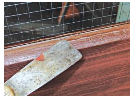
Smoothing new silicone around the glass has left a fine string of surplus material to be removed when cured
