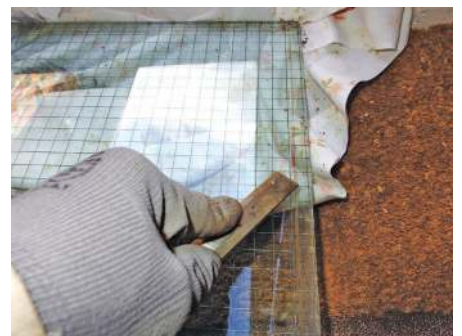
A slightly 'off sharp' chisel being used to scrape off all major surface accretions
