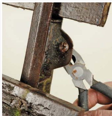
Pliers and a wide blade screwdriver might work, otherwise use a hacksaw
