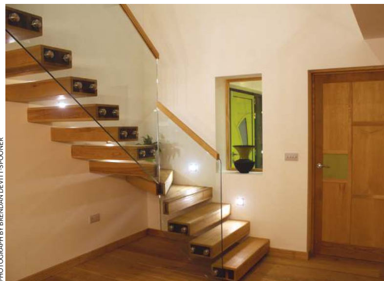
Glass panels finally fitted to the ash-boxed staircase
