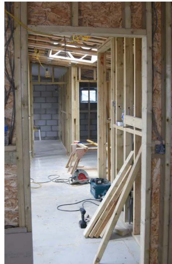
Some of the complex studwork to create the interior room spaces
