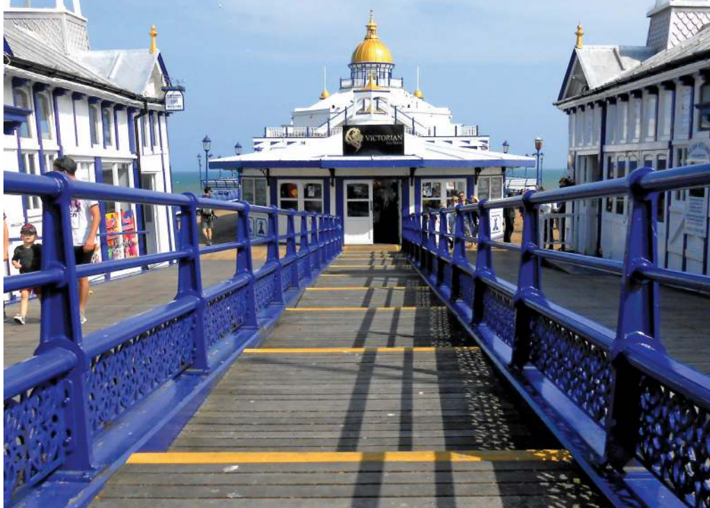
Eastbourne pier – cast iron with timber decking
