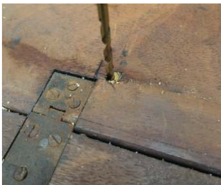
The screw holes were worn out. First some hide glue was squirted in, then a softwood plug inserted, which was then drilled to pilot diameter
