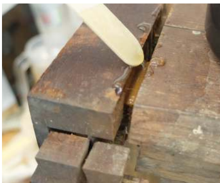
Another joint could be partly separated – one tenon had broken off
