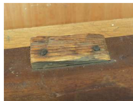
Only one nailed-on wedge present, used to hold a leaf level
