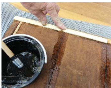
Plenty of glue on the board joints and the new slips added at each side
