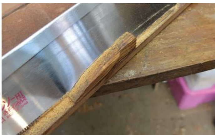
Trimming the leaf wedge at an angle to make it less visually obvious
