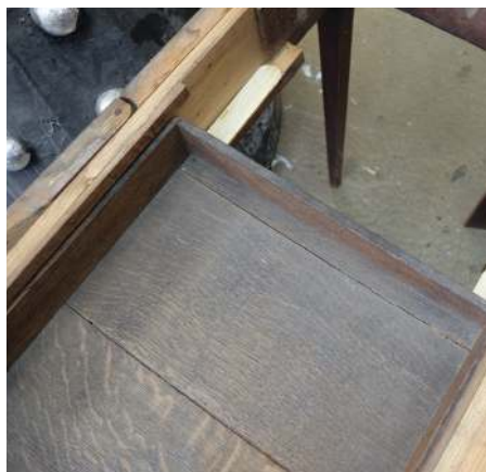
Slips of softwood were tried for thickness prior to gluing
