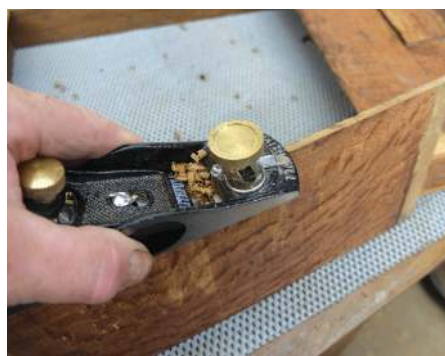
The front board was left in place. The others had their edges planed
