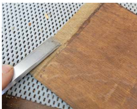
The boards were scraped clean of the remaining glue
