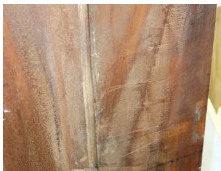
Original cross-grain plane marks on the underside of one leaf
