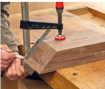
Mark the spline positions
