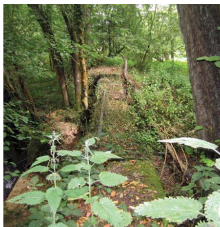
Defunct dam in woodland
