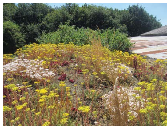
The sedum roof over the main covered area
