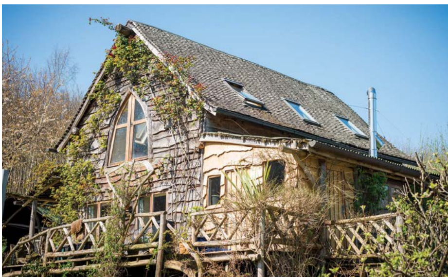
My roundwood timber-frame house, constructed on a framing bed and raised by hand in the woods
