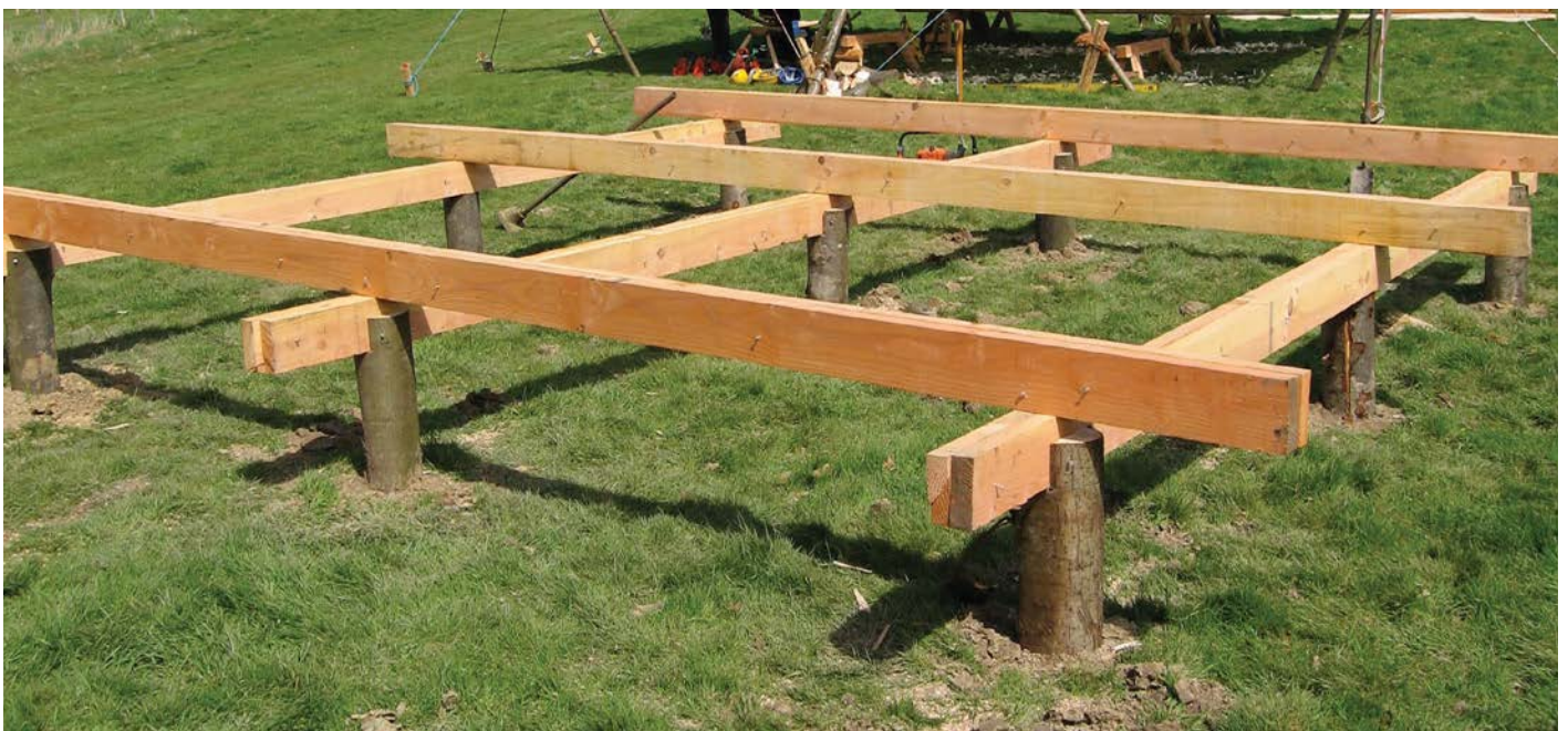
The completed framing bed
