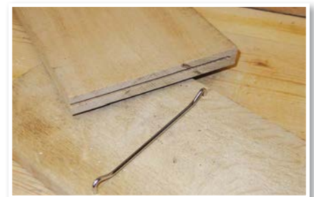
The shelf ends have stopped slots making the magic wire supports invisible
