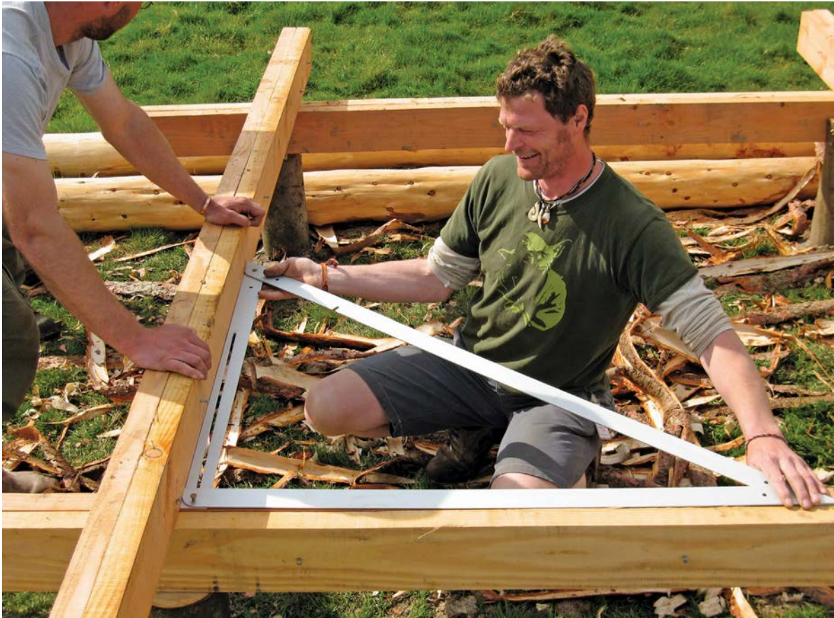
Using the 3/4/5 triangle to get the layers of the framing bed at 90°
