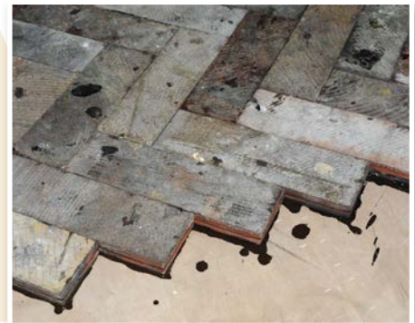
Reclaimed woodblock flooring being laid, which will be sanded once complete
