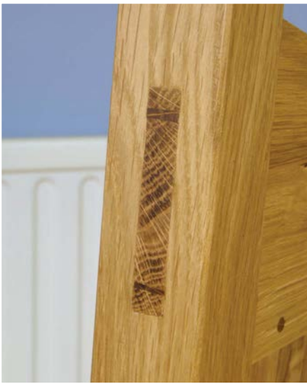
Through-wedged tenon
