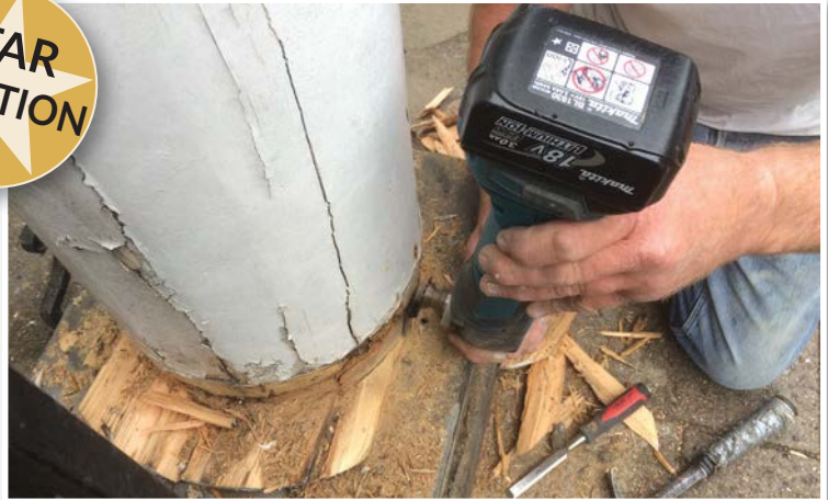
A downward cut with a multi-tool, stopping just short of the lead capping
