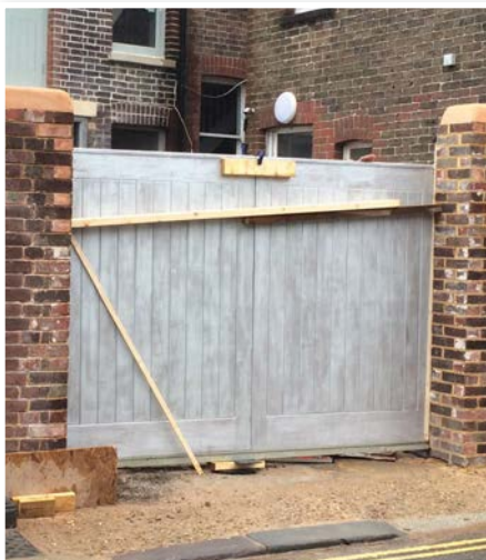
This hardwood gate has been coated with aluminium primer ready for painting
