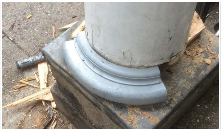
Turned as a ring and split into four segments ready to bond into position
