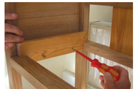
Screw drawer slide support pieces into place
