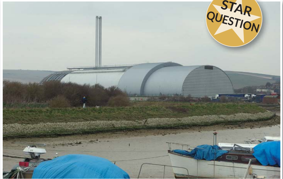
An incineration plant that can produce electricity from domestic waste
