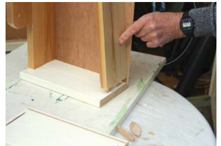
Cut matching biscuit slots to join the sides to the inner front and rear pieces of the drawer
