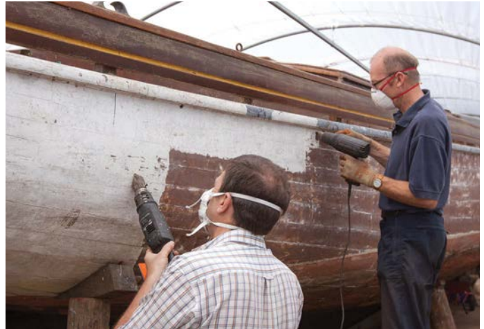
Stripping Olive's hull back to bare wood during her restoration
