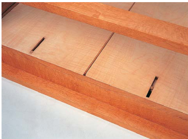
Detail of underneath the top compartment showing peg handles for secret drawer
