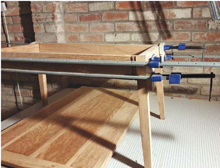
Ensure the sash clamps joints close tightly
