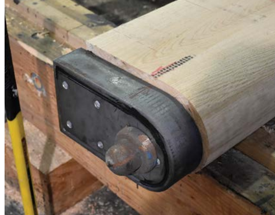
Bottom end of a hinge post with the hinge pin fitted
