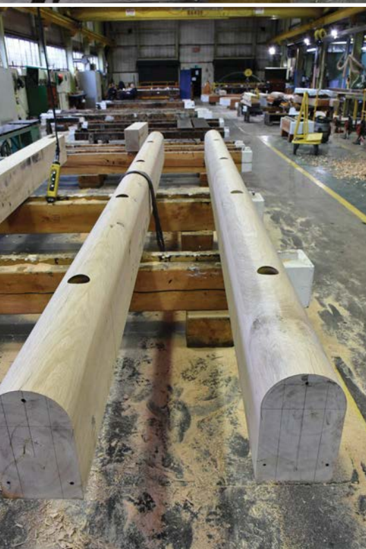
Two hinge posts with borings for steel rods
