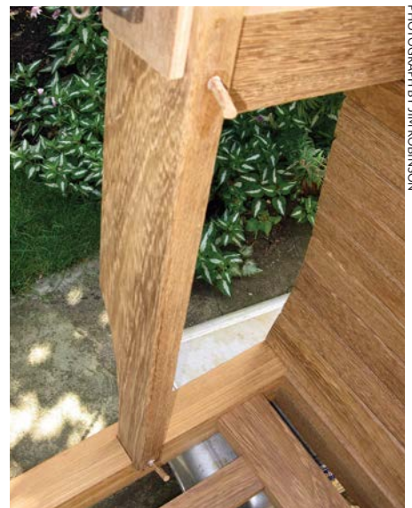
The teak dowel tapped into the chair joints
