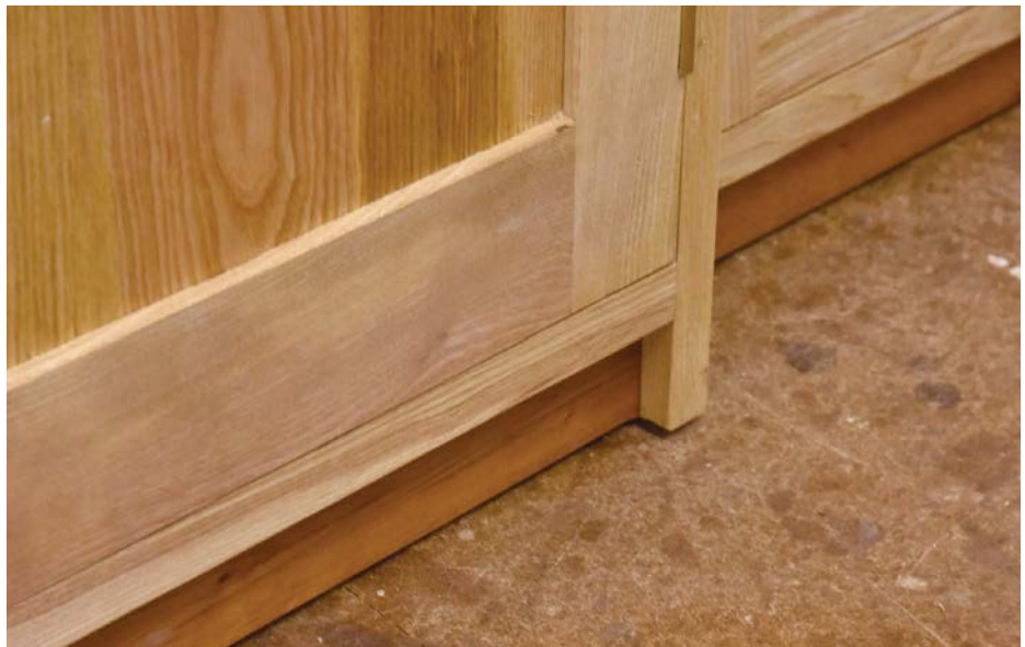
Breakfront detail at floor level
