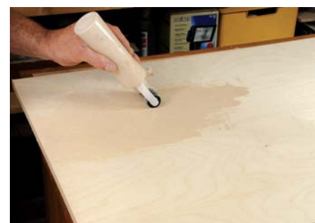
An alternative using a roller to apply aliphatic resin for pressing
