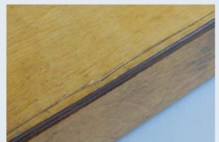
Top surface of the broken rule joint on the leaf
