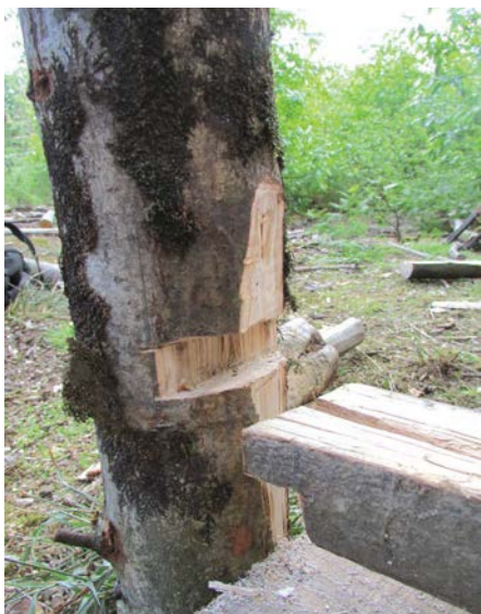
The tongue ready to insert into the slot
