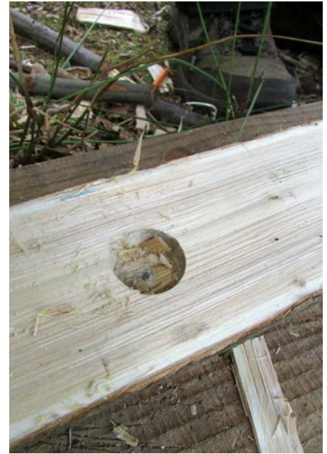
Hole drilled for a zale in the bottom rail
