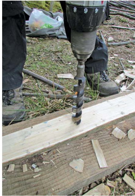
Drilling out holes for the zales using a cordless drill and a 1in (25mm) bit
