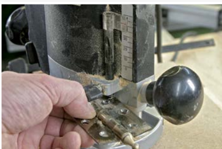
Checking the thickness of a hinge to inset it into a stile
