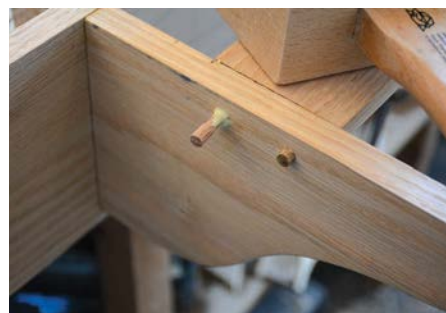
The peg rail can now be drilled and dowelled in place
