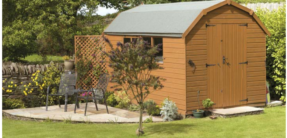
A large garden shed dedicated to workshop activity can be surprisingly roomy
