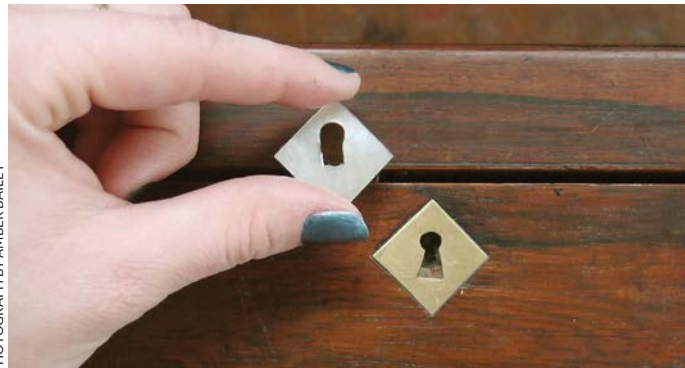
An original worn piece of mother of pearl inlay replaced by a new brass escutcheon
