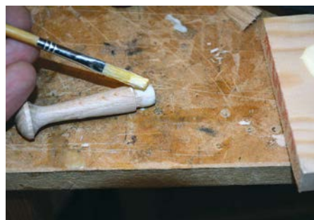
The peg ends are lightly brushed with aliphatic resin glue
