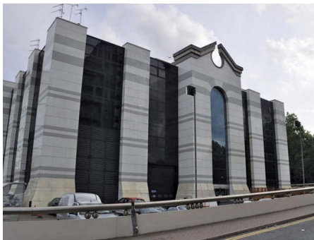
The now-demolished Marco Polo building in Battersea, South London – an example of Post-Modernist architecture
