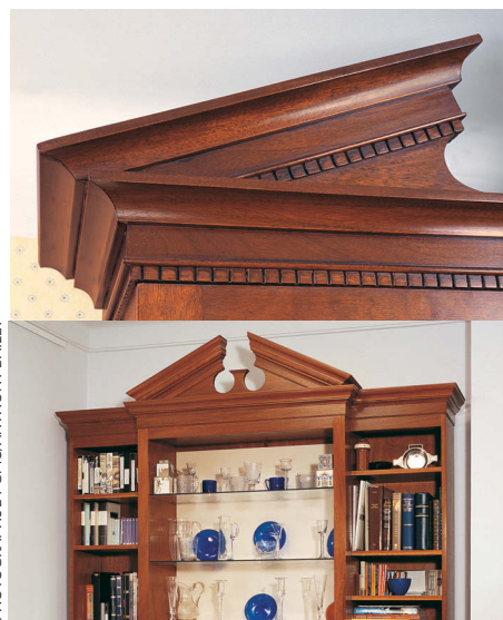
Top: A broken pediment with cavetto and dentil mould details on top of a large mahogany bookcase
