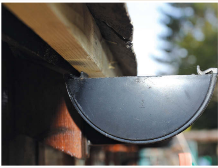
Eaves meeting the gutter
