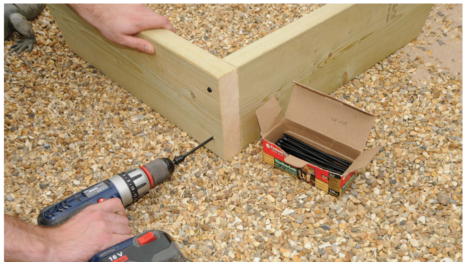
For some outdoor tasks, such as decking assembly, exterior adhesive is completely unnecessary, especially if using dedicated timber screws
