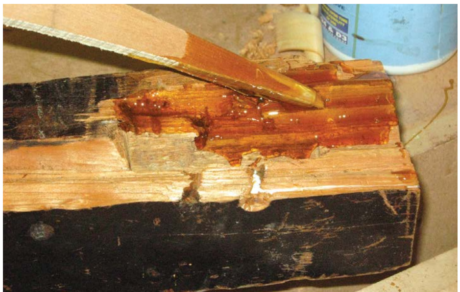
PU used for a gap filling repair
