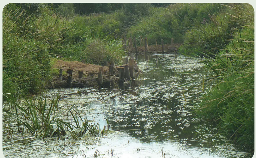
Creating river bends using willow to slow water flow
