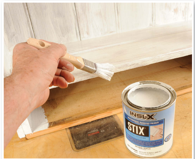
Very difficult surfaces, such as this pine which has wax ingrained into it, may need a special bonding primer like this one
