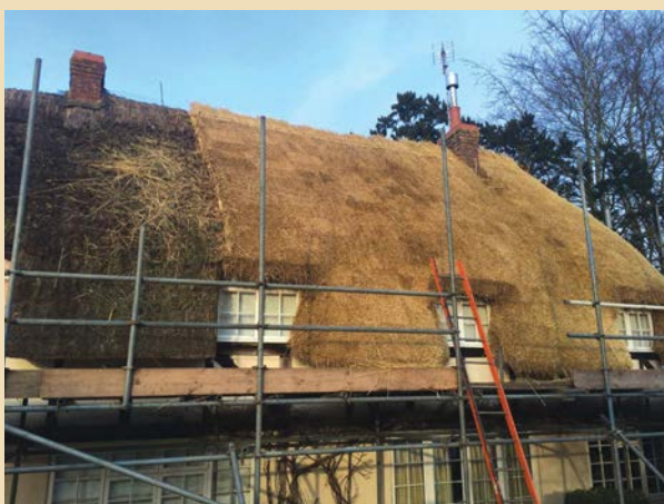
Total re-thatch – This cottage in Stockbridge, Hampshire has been re-thatched in traditional wheat reed and finished in a flush ridge. Top: Before work began; Above: work in progress; Right: the end result. The main coat work will last for at least 20-25 years, but would require some attention to the ridge in 10 years or so
