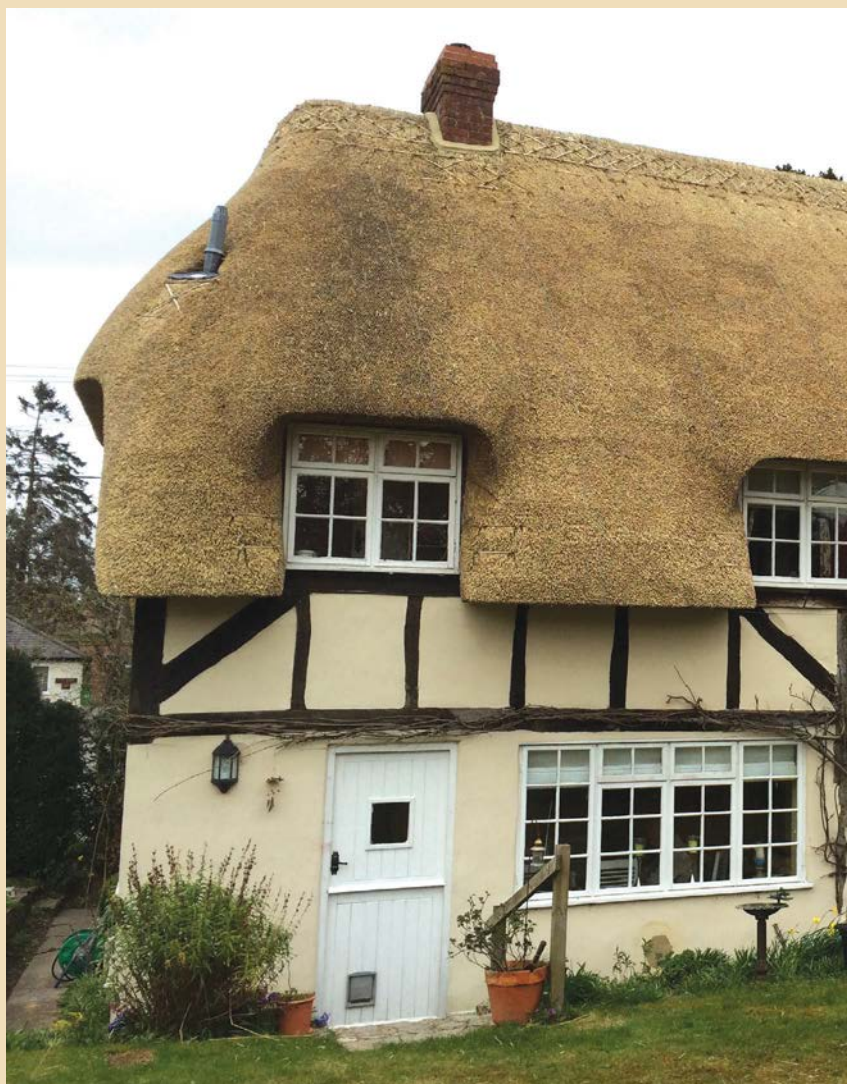
Total re-thatch – This cottage in Stockbridge, Hampshire has been re-thatched in traditional wheat reed and finished in a flush ridge. Top: Before work began; Above: work in progress; Right: the end result. The main coat work will last for at least 20-25 years, but would require some attention to the ridge in 10 years or so
