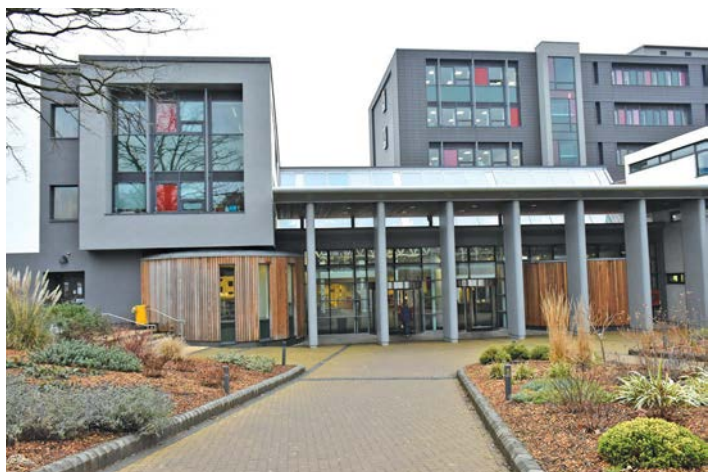
Left: Warwickshire College's front entrance with new facade Right: Ziricote veneered table
