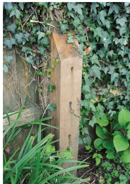
An oak spur used to extend post life
