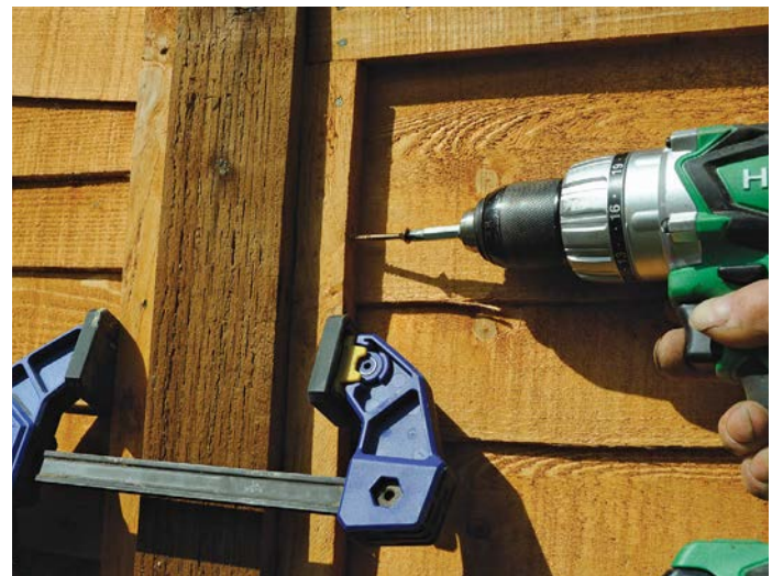
Clamp and screw panels to posts
