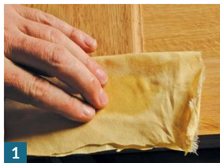
1 Apply a wetted cloth to the damaged area
