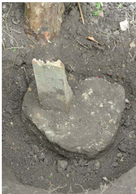
Removing concrete is a real nuisance
