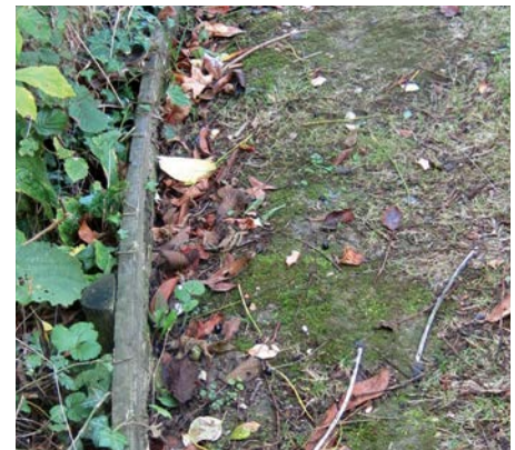
Small revetment by path
