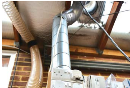
Rigid ducting is more efficient
