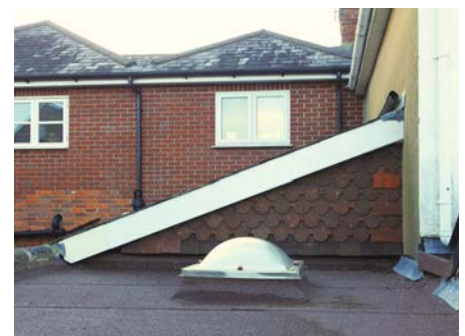
Fitting this uPVC bargeboard was a 30 minute job, safe working access to the roof is key though
