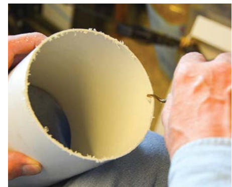
De-burr to eliminate snagging points
