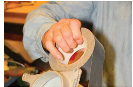
Make pipes airtight with tape
