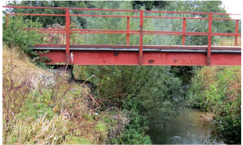
River Uck, gabions rock filled cages by bridge – spile banking beyond
