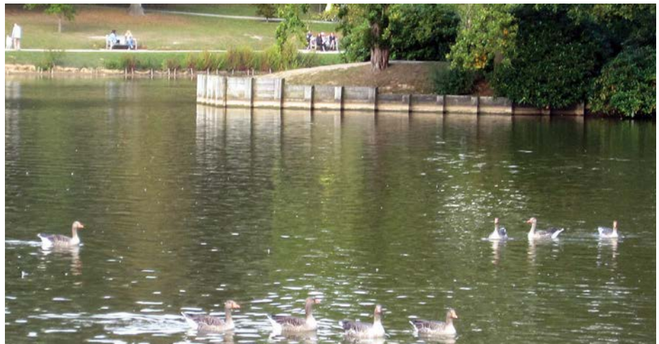
Larger scale revetments
