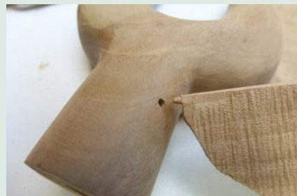
Repair of woodworm hole
