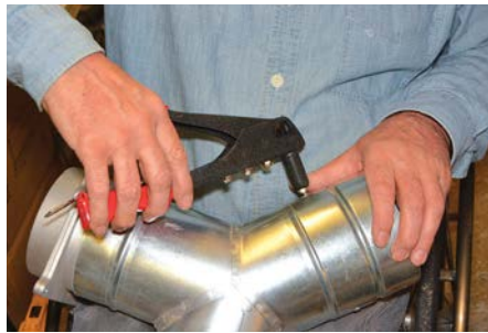
Secure pipes with pop rivets
