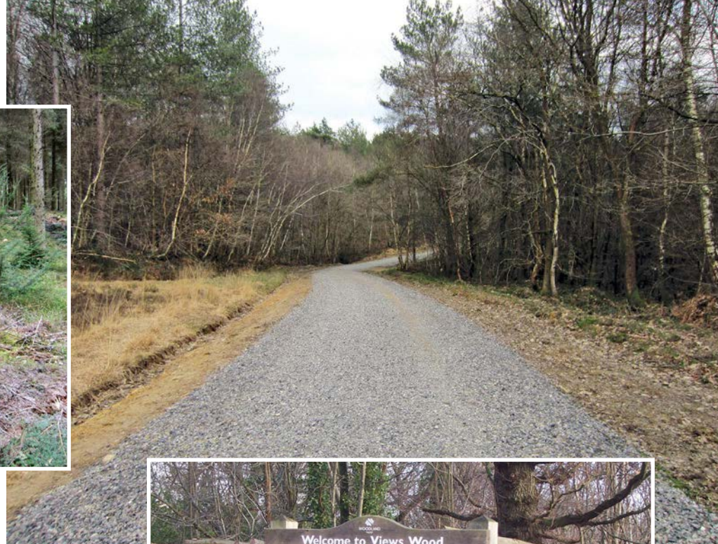
Above: A fully engineered forestry access track
