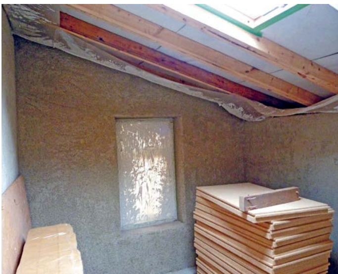
Hemp lime plastered walls in the bathroom with wood fibre blocks to be used to insulate the ceiling
