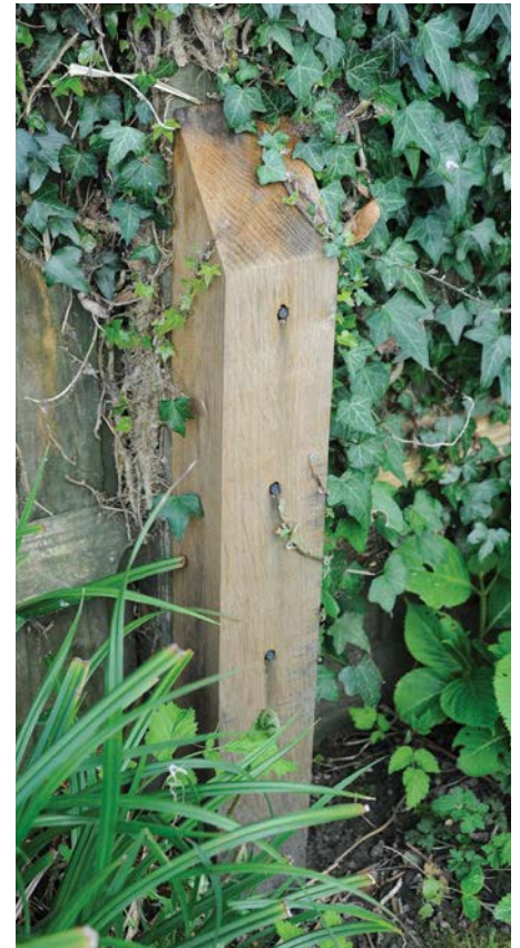
An oak stub post has been used to extend the life of a softwood fence post
