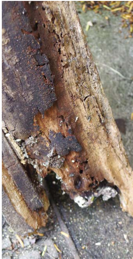
The rotted underside of a door sill soon becomes a home to a variety of organisms
