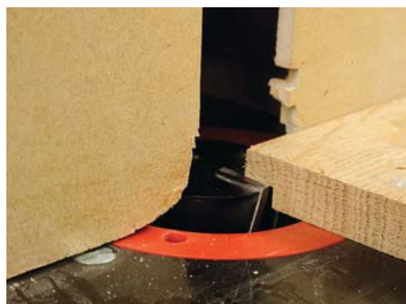
The panels are rebated to sit in the bed frames
