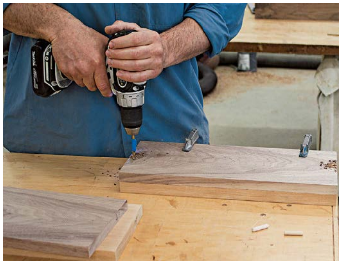
When facing the wood for the stiles, drill for ¼-in. dowels through each end to help keep the material from slipping during glue-up. Apply several clamps around the perimeter for plenty of holding strength as the glue dries
