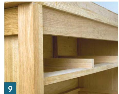
The back panel allowance – shown on the finished piece
