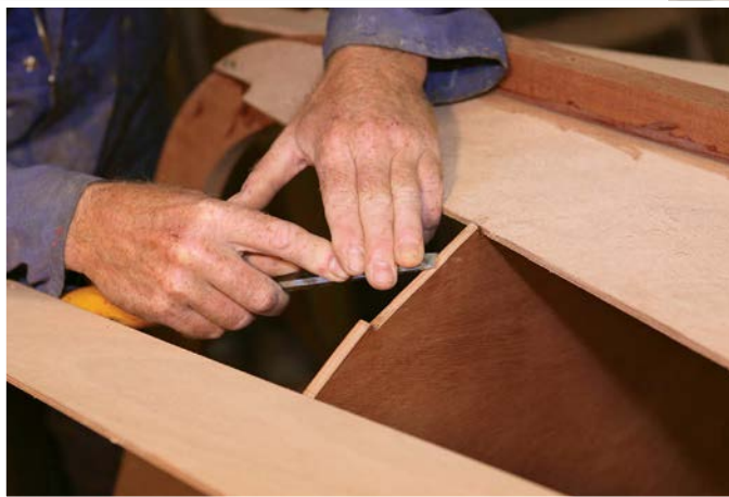
Each step has to be trimmed slightly so the next plank fits snugly in place
