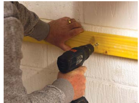
Then I used a masonry bit to drill and mark the blockwork through the wood
