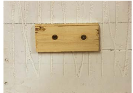
Temporary support blocks were used to rest the frame on for pilot hole drilling
