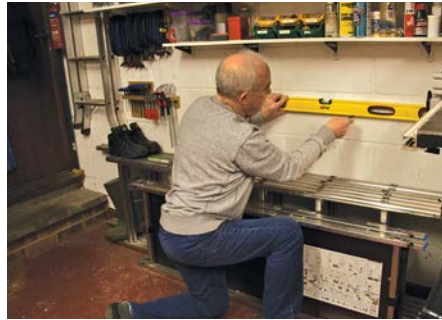
Marking up the wall, avoiding the mortar line so the bolts would anchor properly
