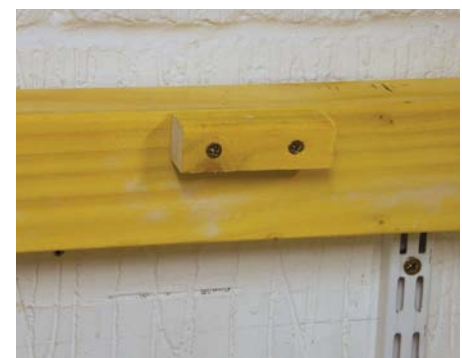
Blocks were screwed on for fixing the top down with vertical screw going up through each one
