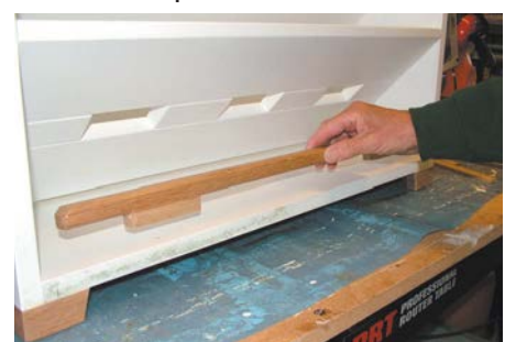
Positioning the oak retaining rail
