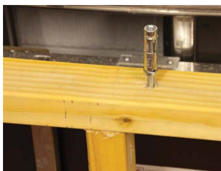
All the anchors were pre-installed in a line ready to push home in the blockwork
