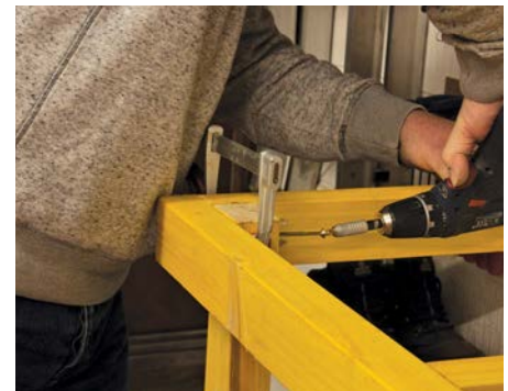
A leg clamped in position and drilling to take standard twinfast screws
