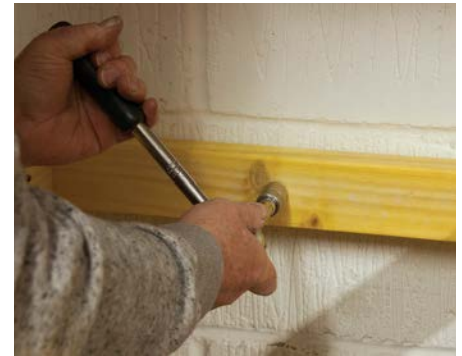
Using a ratchet wrench and a socket of the correct size to tighten the anchors
