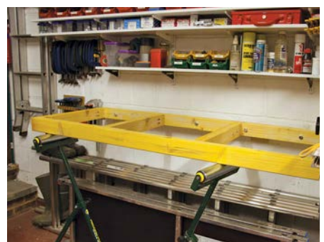
Two roller stands kept the frame level during wall fixing
