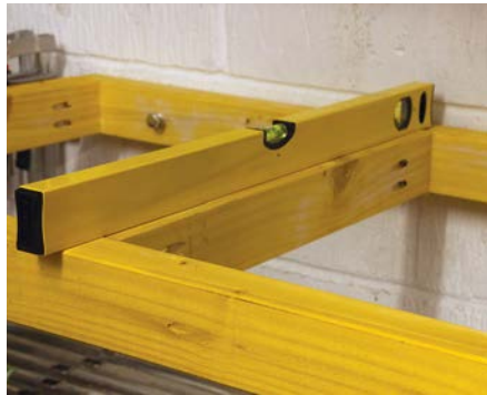
Checking for level before tightening the anchor bolts
