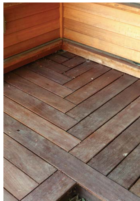
Right: A Herringbone pattern is an attractive way to intersect two sections of decking that have perpendicular deck boards. Here, the picture frame on the right becomes part of the deck pattern on the left.
