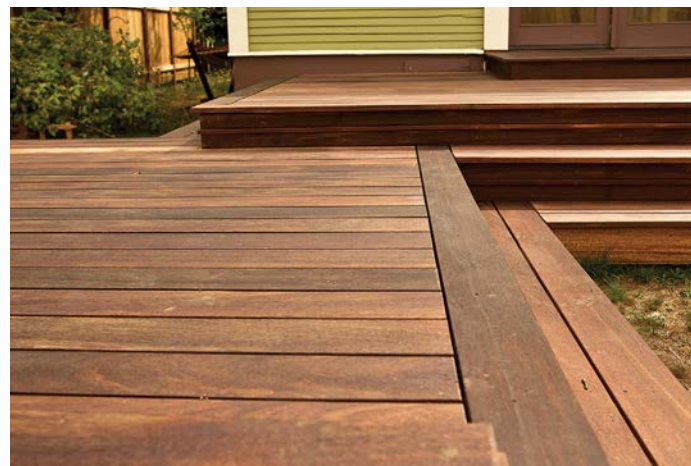
Above: A picture-frame border runs perpendicular to the field decking. On this deck, the borders visually tie together the deck and wrap-around steps.
