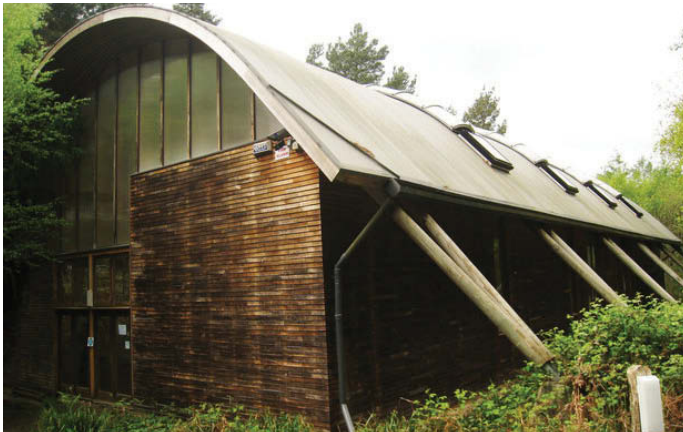
The Woodland Enterprise Centre at Flimwell, East Sussex
