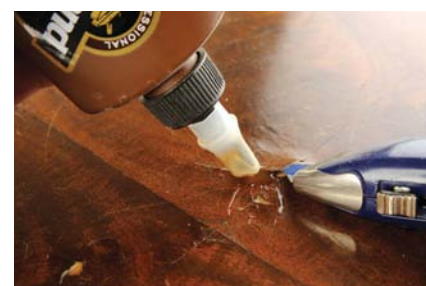
Using readymade hide glue under the repair then pressed down firmly
