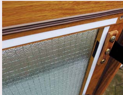
The coated steel self-adhesive strip in position, the magnetic strip is stuck to the polycarbonate sheet
