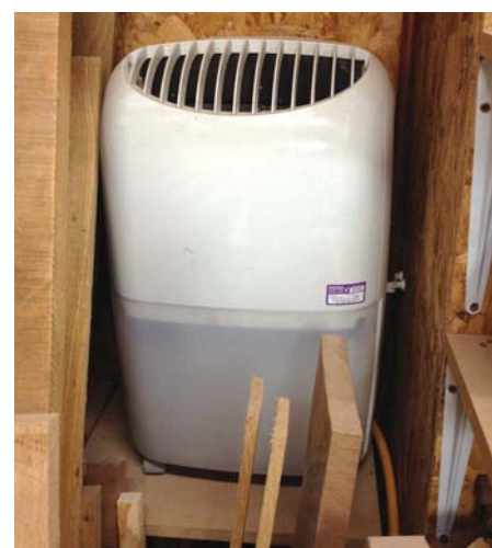
Our plumbed-in dehumidifier drying the timber
