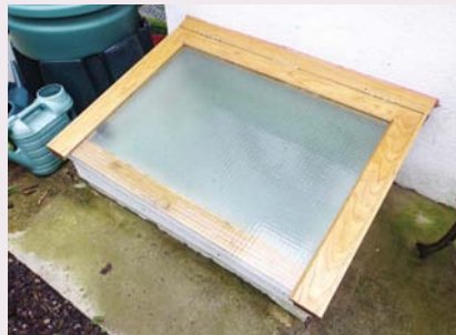
The fanlight ready for more cold condensation forming weather
