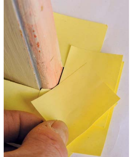
Use plenty of post-its to fit the profile
