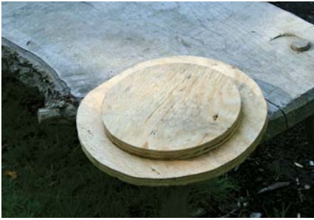
A plywood bung seals the steam box
