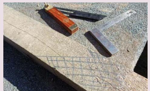
Above: Marking out the scarf
