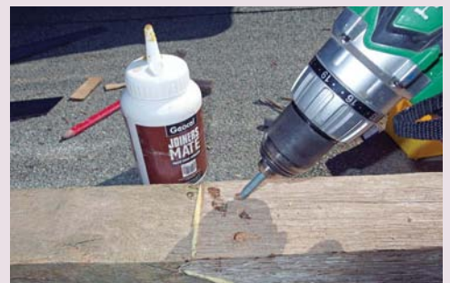
Below: Drilled, glued and screwed
