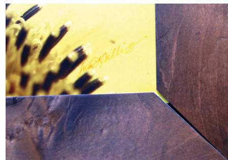
Mitre joint on a picture frame held with only glue
