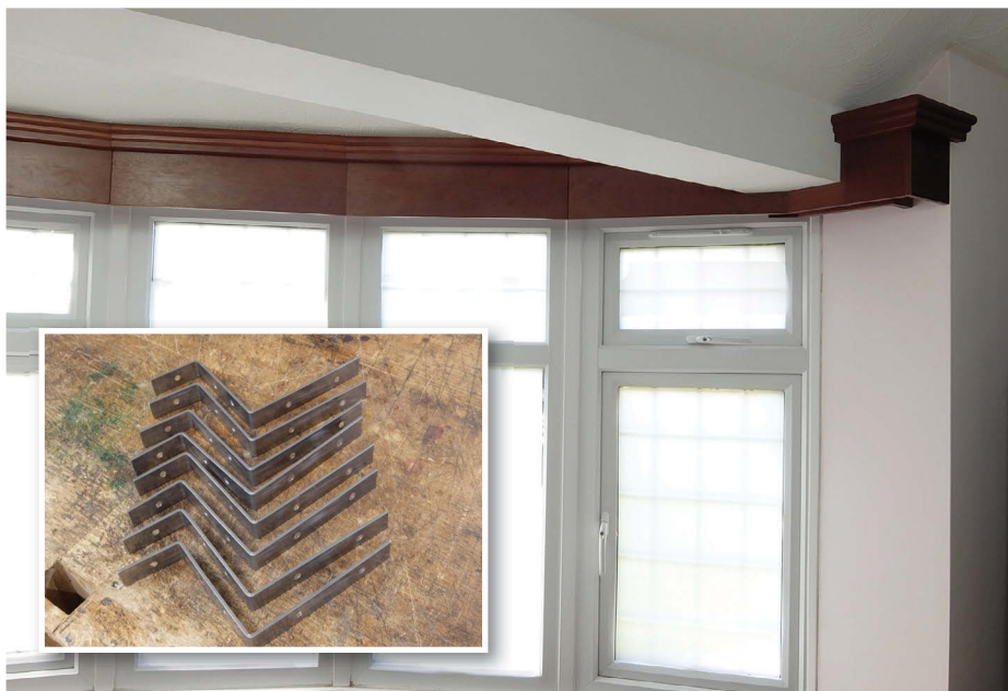
The shaped pelmet fixed in position and finished Inset: The brackets for the fixing of the shaped pelmet
