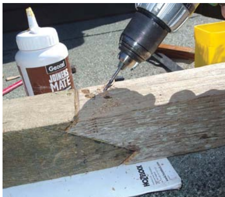
Repairing a fence post using a zig-zag shaped scarf joint
