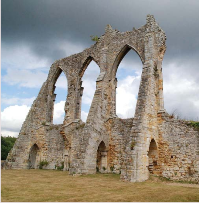
The ruins of Bayham Abbey works well as an image for its very distinctive architecture
