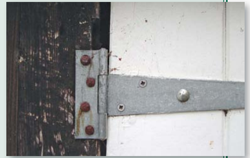
Rose-nailed strap hinge with coach-bolt through door
